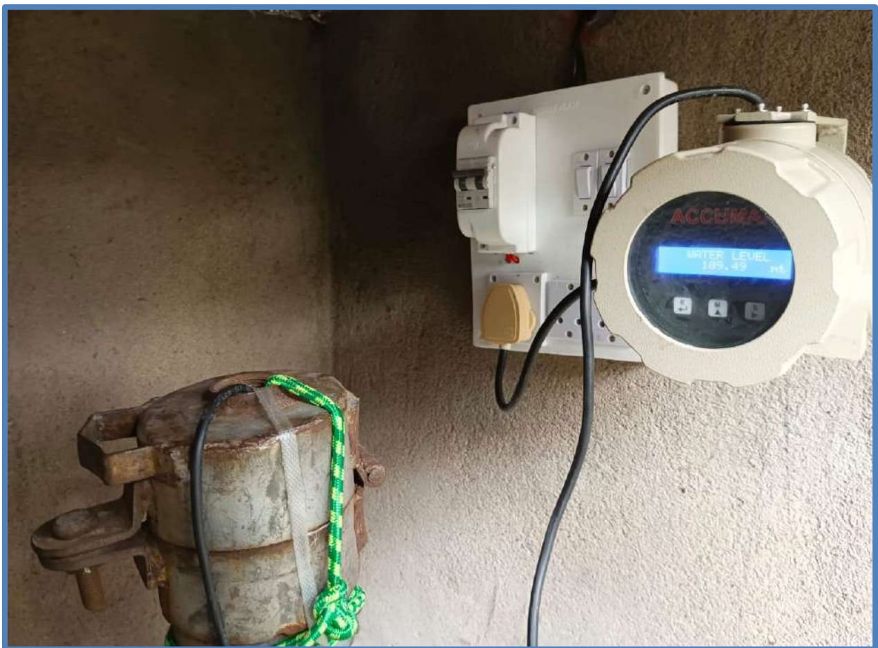
Picture 12 – Piezometer well
