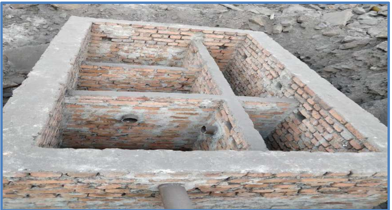
Picture 10 – Oil & Grease Trap
